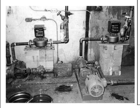
This picture shows the piping used to transfer resin from storage tank to various mixing tanks in a paint factory. Notice the motor pumps, flow meters, various valves and the threaded carbon steel piping. The supports and layout of all components was dictated by cost constraints.
